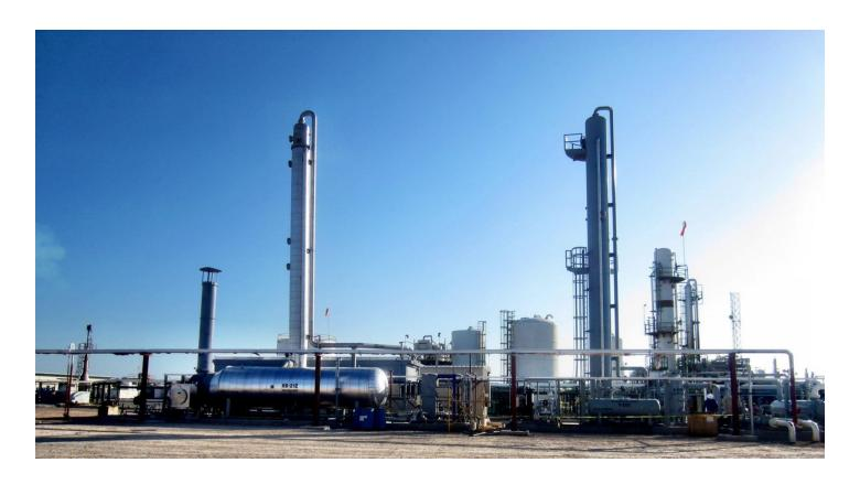
Finally, once the CO2 is separated, it is compressed to extremely high pressure and prepared for sequestration.
