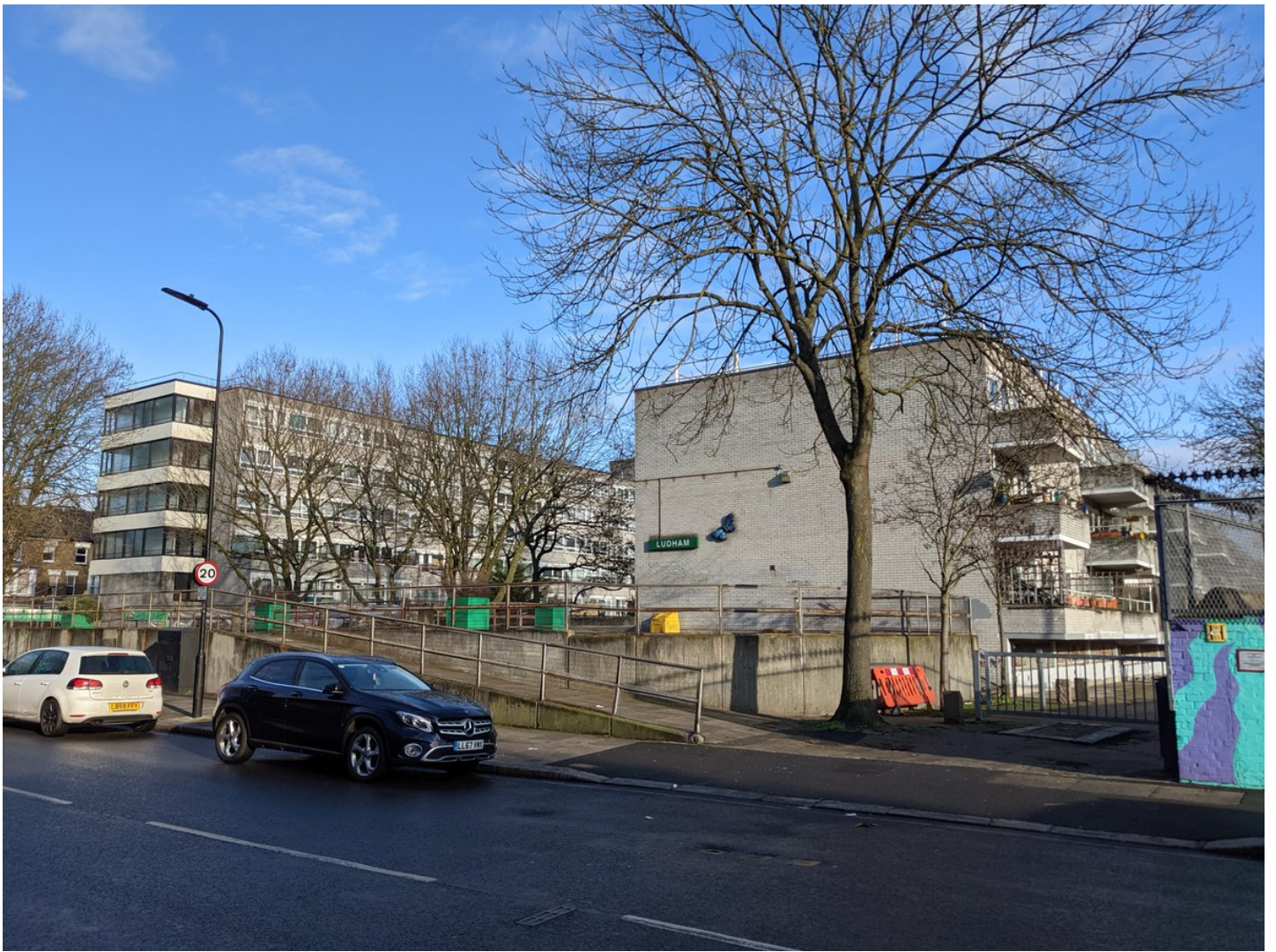
13/ The Mansfield Road Estate, 73 flats and maisonettes, designed by George Benson and Alan Forsyth of the Borough Architect's Department and built 1974-1980.
