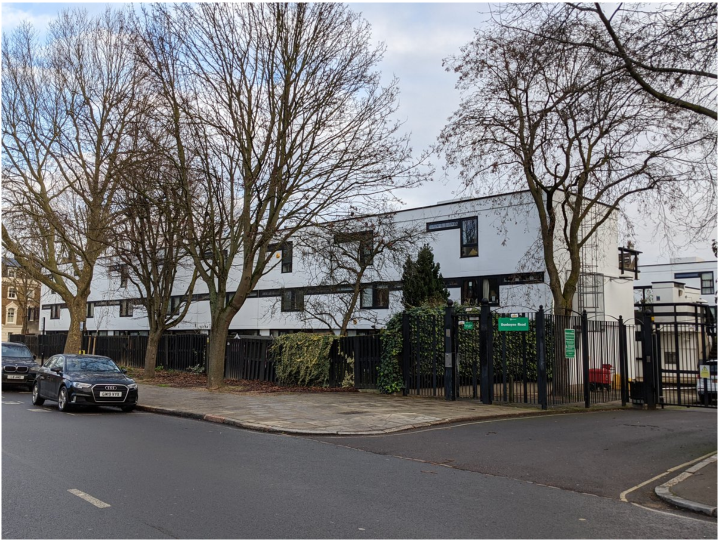
12/ The Waxham and Ludham Estate designed by Frederick MacManus & Partners for the Borough and built 1974-79.
