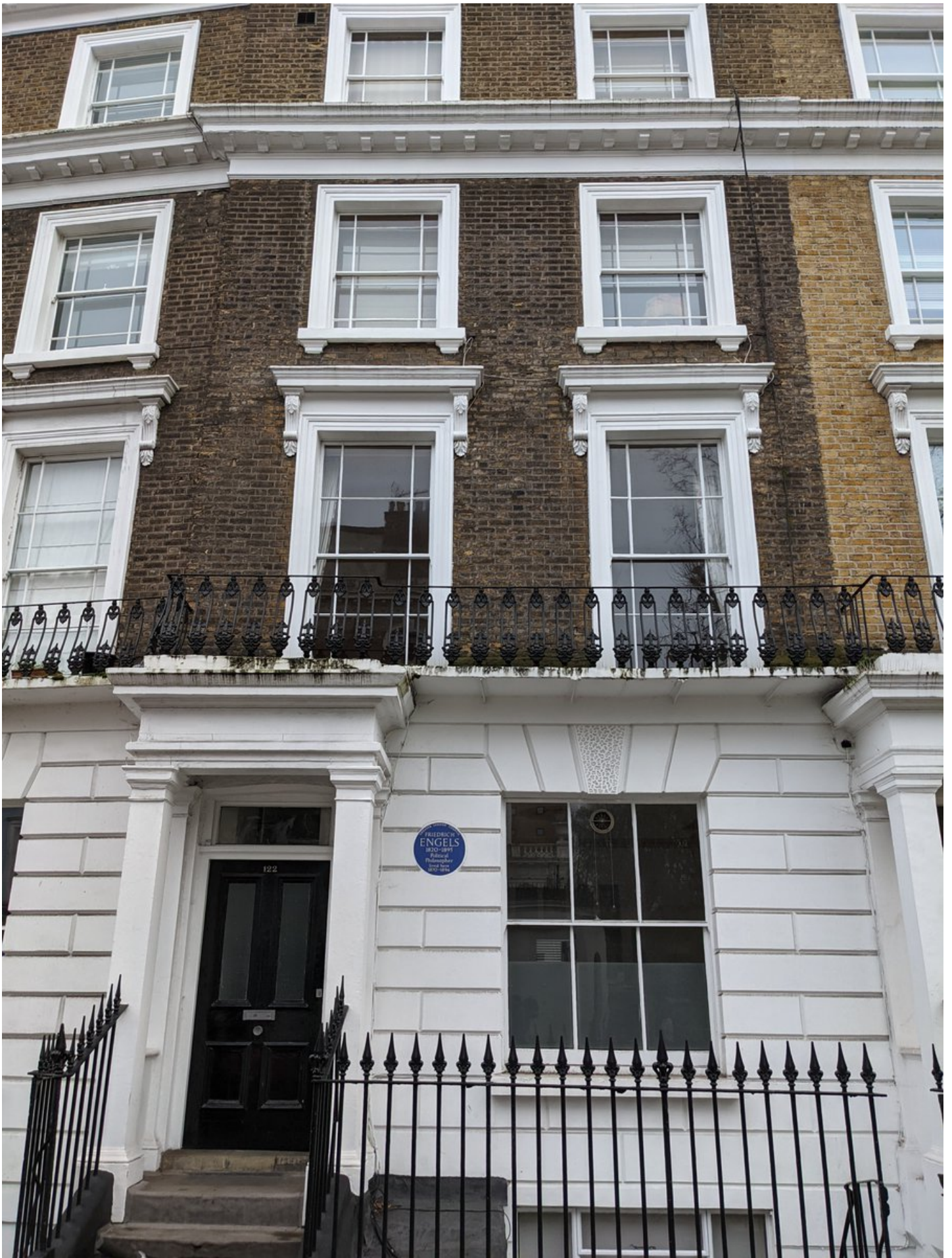
8/ Constable House, a four and five-storeyed neo-Georgian balcony-access tenement block, designed for the London County Council by Louis de Soissons in the early 1950s.
