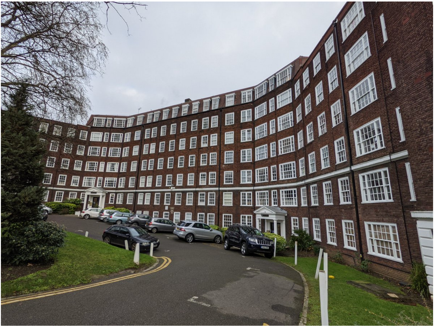
10/ Barn Field and Wood Field built in 1947-9 for Hampstead Metropolitan Borough Council and designed by Donald Hanks McMorran. Grade II-listed for their 'combination of Soanic and Scandinavian devices, producing a lean, spare but exceptionally well-proportioned classicism'.
