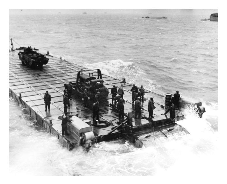
The Great Storm forced revision to the LST to rhino to beach plan, as many Rhinos suffered serious damage and performed poorly in rough weather.
