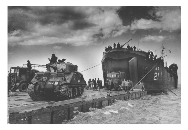
The real trade off in adopting direct beaching of LSTs as the norm was the increased number of damaged ships, but the Admiralty came to approach of the move as it allowed much faster unloading - and LST repair turn around was much better than feared. /11
