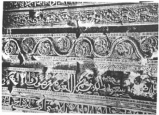
43. A panel of the so-called Kutub tower in Delhi. The exquisite serpentine Hindu pattern in the upper part is the wreath called 'Makar Torana' because it emanates from the mouth of a crocodile. This is a very common sacred Hindu motif in historic buildings. The Islamic tampering and forgery in stone may be seen in the lower portion. An attempt has been made to plant Koranic lettering. Such forgery in stone fooled even historians who thereby inadvertently ascribed these buildings to Muslim authorship.
